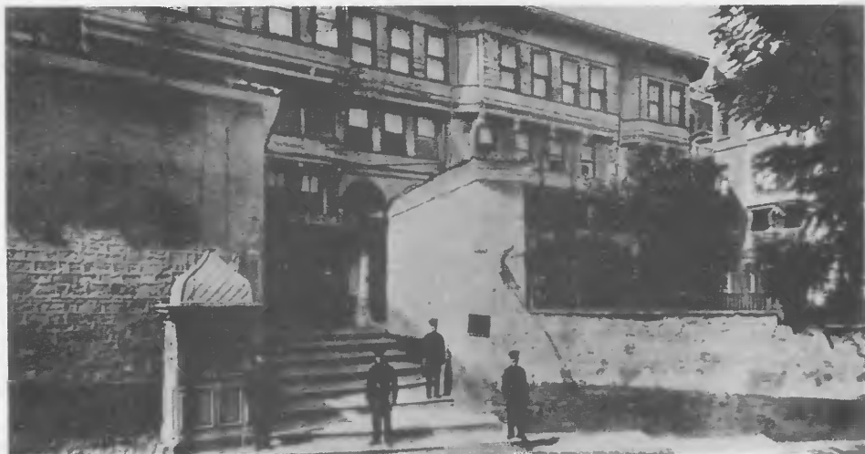
Gate entrance to Ecumenical Patriarchate at Phanar and building before destruction by fire in 1941.
